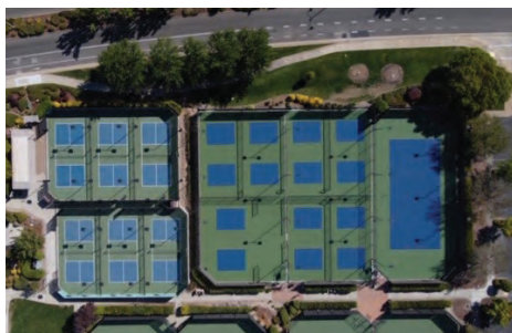
Courts in Progress, Photo by Tom Peach
