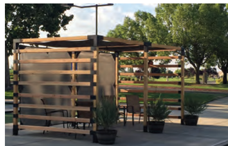
Enhanced Shade Structure
