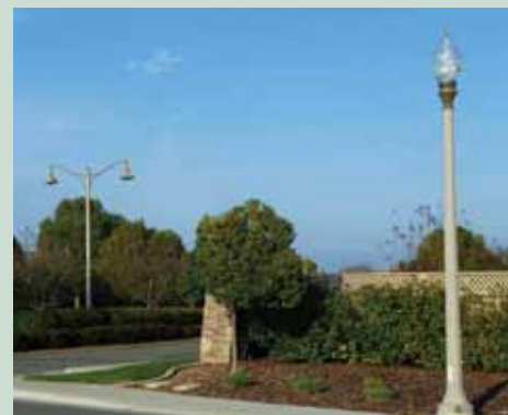
Existing pendant streetlight on main roadways (left) and "acorn" light in neighborhoods
